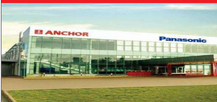
Anchor by Panasonic Location : Bhuj, Gujarat
